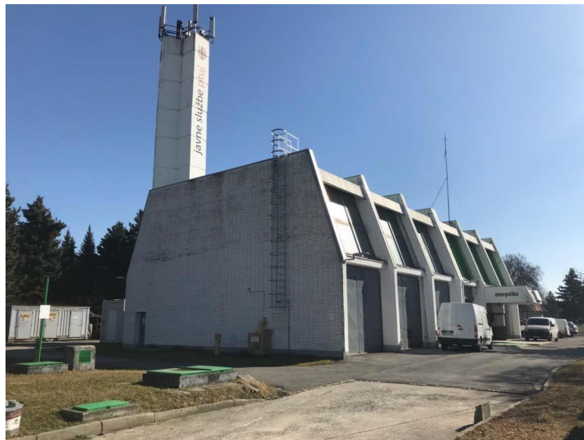
Obstoječa kotlovnica zunaj
